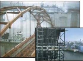
Engineers from around the world watched as Simplex hollow hole cylinders raised a 6,000 ton bridge section more than 170 ft. over the Willamette River in Portland, OR. The span was constructed up river and barged into position. Using pull rods and couplings, Simplex RCD200 Series cylinders completed the lift in 40 hours.
